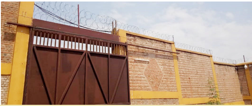
High wall at Nyarugenge correctional facility with concertina wire around the fence to prevent possibilities of escape
