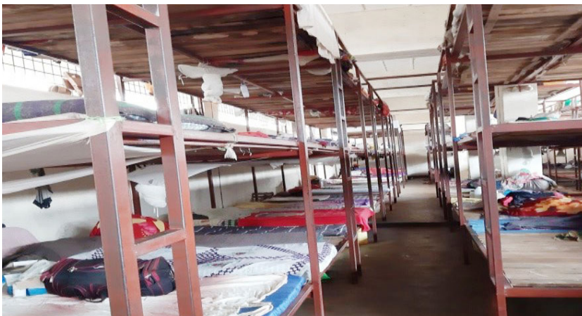
Huye new building named "turwubake" block that tends to comply with rule 12 (accommodation) of Mandela rules
